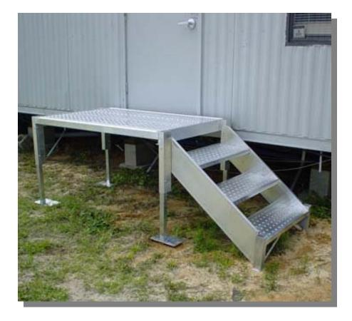
4. Bring system flush to building so platform is level with threshold
